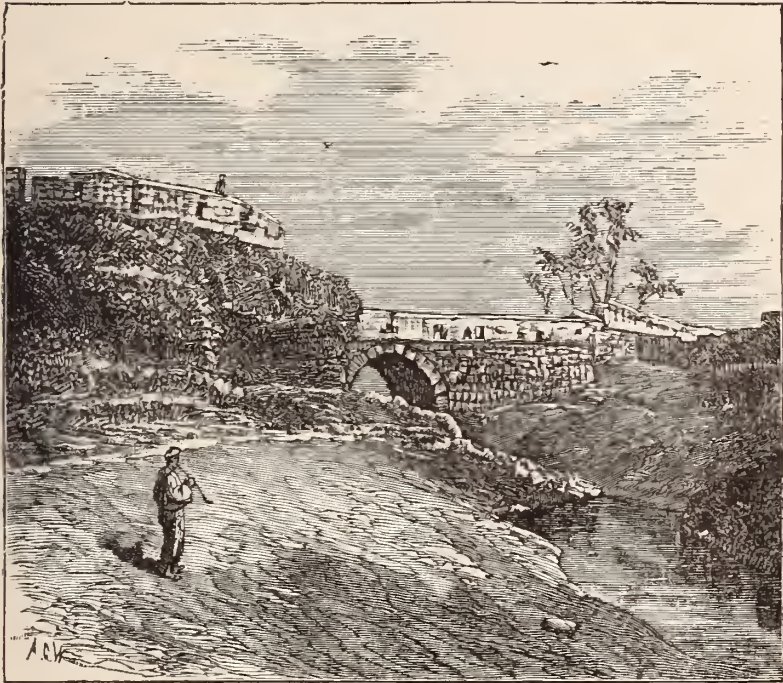
The Walls of Seoul (from a Photograph, 1876).
